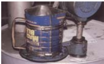
Open Fluid Containers
